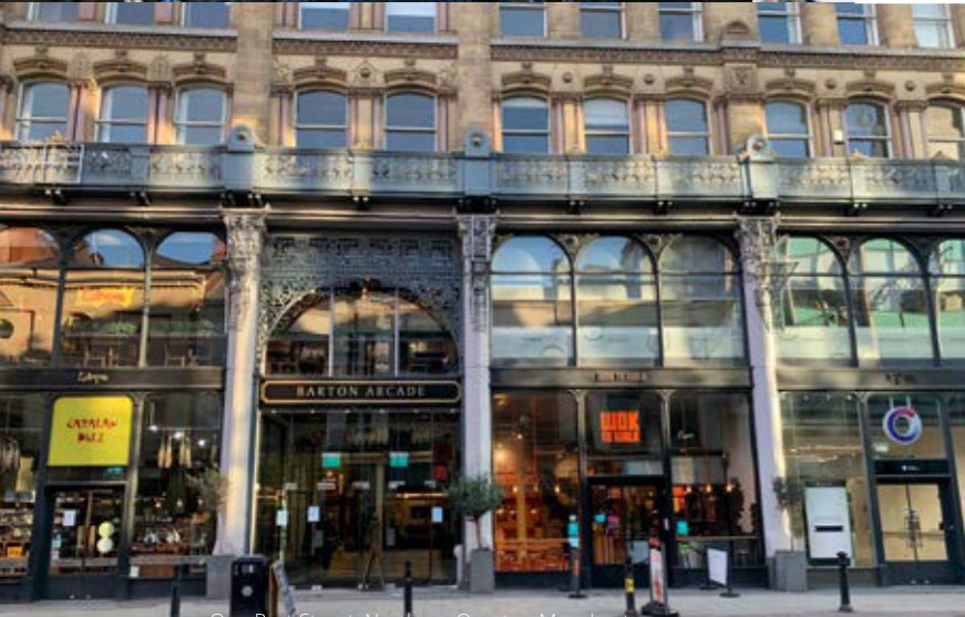
One Port Street, Northern Quarter, Manchester
